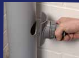
3. Insert Easy Boss into hole
