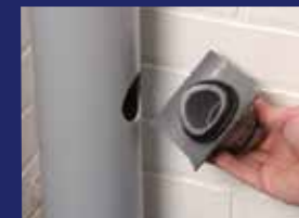
2. Ensure seal is in position
