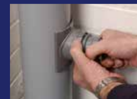
4. Twist in the Easy Boss connector
